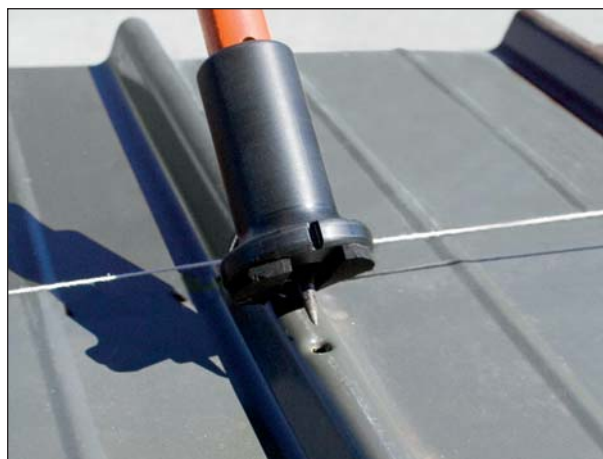
Perforation \varnothing 8 mm
